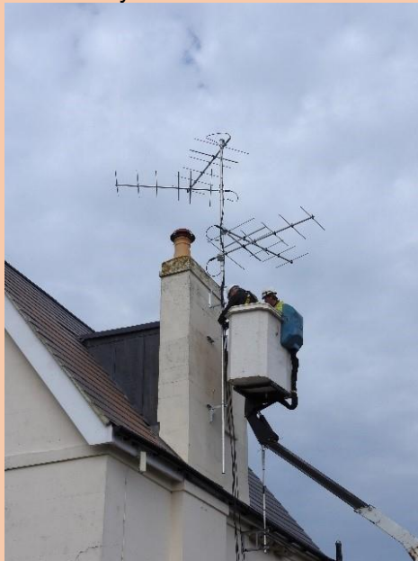
Installing the antennae and the control box
